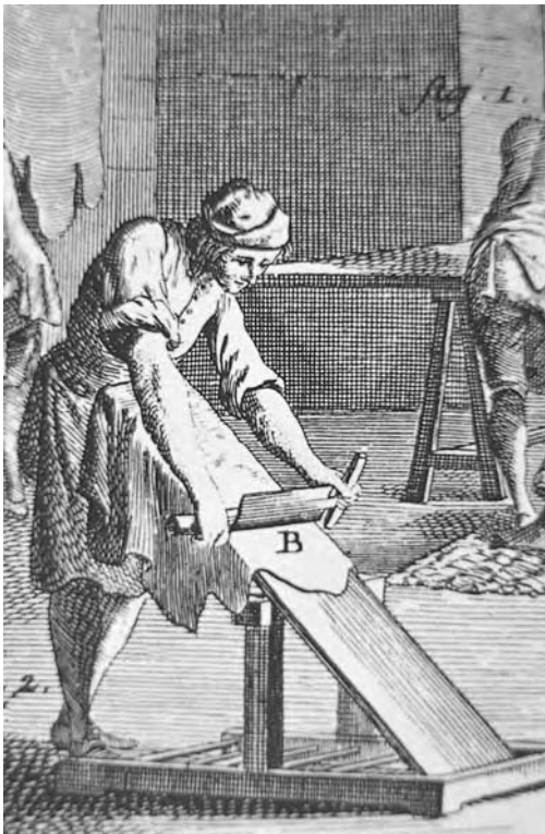
Figure 7.7 Shaving leather to uniform thickness.
